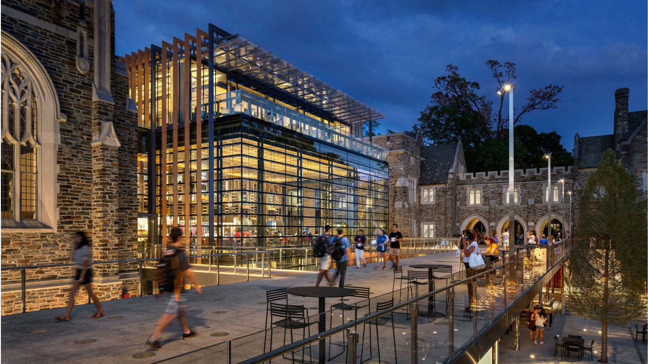
West Campus Union, Durham , North Carolina by Grimshaw's – ' a glazed social hub in historic city centre' Allowing the university to dominate the area or a genuine attempt to open up the university
